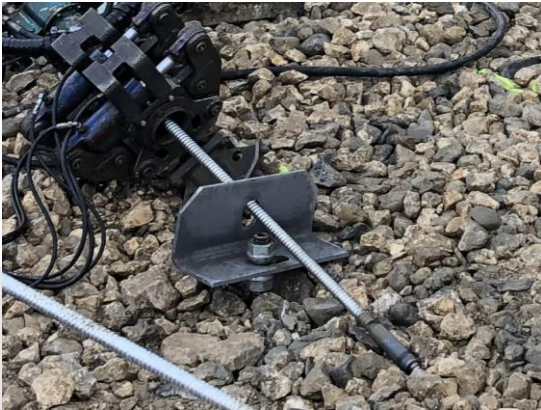
Platine support micropieux
